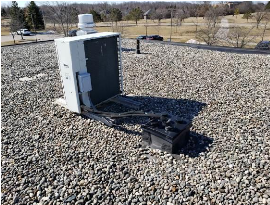
21. Localized HVAC unit on wood sleepers. Should be able to be raised a few inches to sit on newer sleepers and pads with the new roof system.
