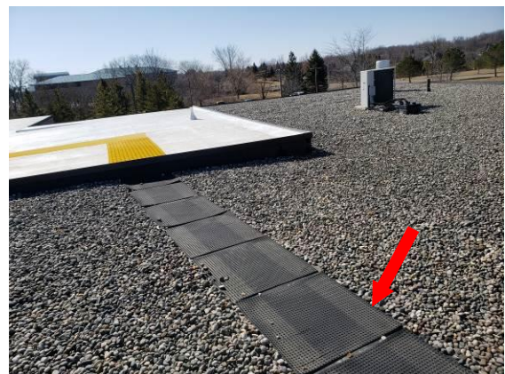
24. Typical existing walk pads. With replacement roof new safety yellow walk pads could be installed, similar to those installed in 2008.
