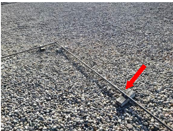
17. Another view of the existing conduit and conduit supports on the ballasted roof. With the replacement roof, newer style supports could be added that may be better systems than simple wood blocking supports.
