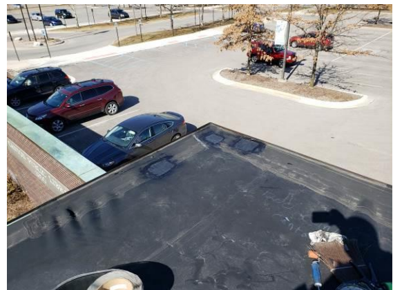
4. Intertek installed repair patches over these holes.
