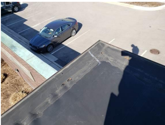
3. Holes found in the NW corner of the east area. The wood blocking at the edge visible through the holes.
