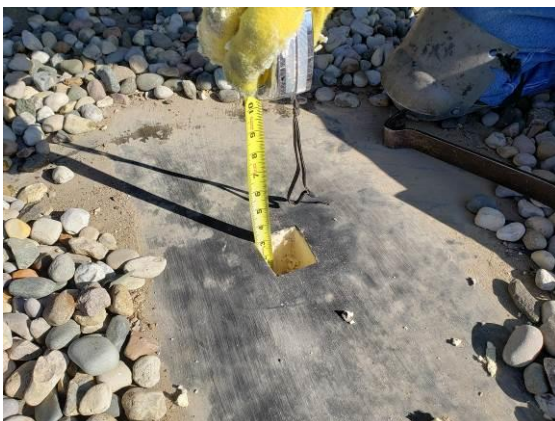
5. View of a typical core in the main roof areas. A single layer of 3" thick rigid isocyanurate foam found over a steel roof deck.
