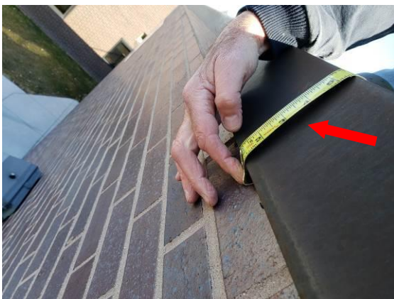
23. Close up measurement of the existing metal. Existing metal is slightly out from brick and is approximately 5 inches in face dimension.
