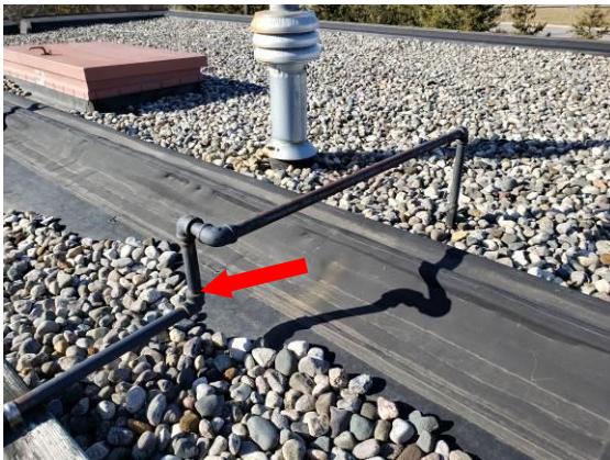
15. Most gas and/or electrical conduit is high enough to remain. Some areas may have to be lifted, depending on the thickness of the recovery insulation.
