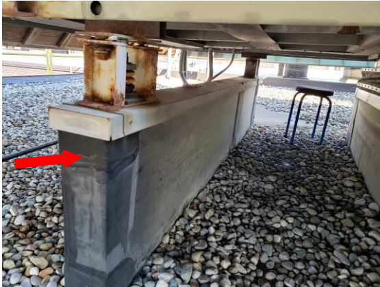
13. View of equipment sleeper supports. Reroofing should be possible without having to lift the large units.
