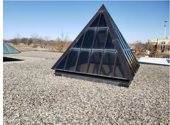
14. An existing pyramid skylight. This skylight should also be able to be reroofed without having to lift and reset the skylight and frame.
